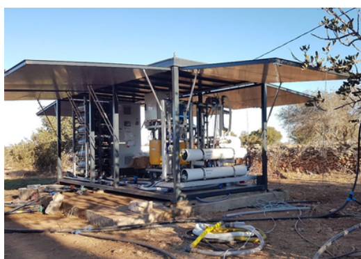
Smart-Cube - pilot-scale plant for the solar-powered groundwater desalination for irrigation by means of MCDI and LPRO (open). Location: Essaouira, Morocco.
