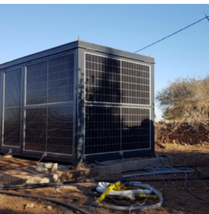
Smart-Cube - pilot-scale plant with PV panels (capacity of 7.6 kWp)
